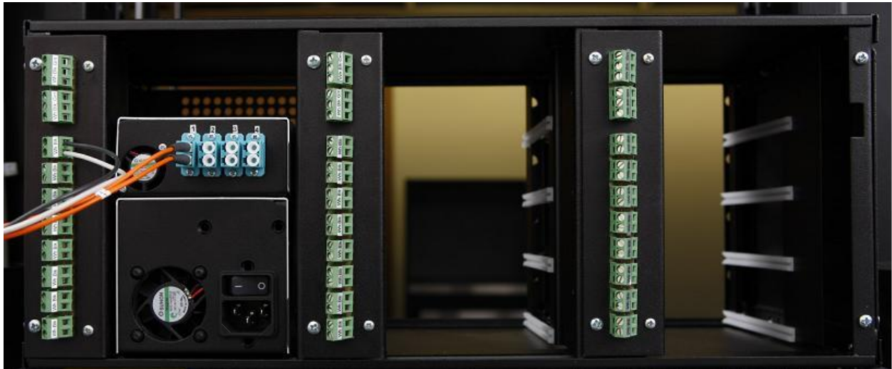
PPP with 1 power supply installed and 1 st media converter module installed. Hybrid cable connects 2 fibers (LC connectors) and 2 copper conductors (via terminal blocks) to transmit data and power for PoE to the remote end.
